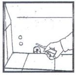
10. The WC pan Should be fixed to floor by screwing it.
